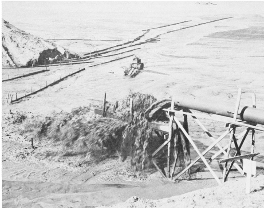
Figure 12 - Hydraulic Fill Being Discharged (Corps of Engineers 1985)
