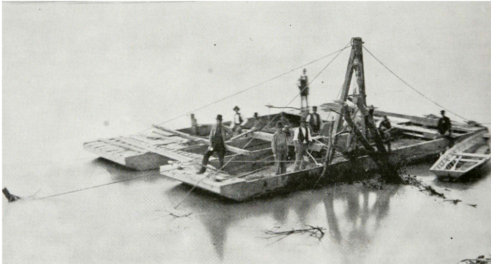
Figure 6 - Typical Snag Removal Outfit (Branyan 1974)
